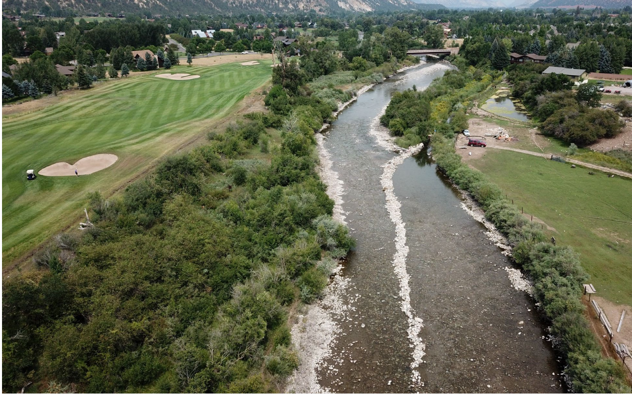
Summer 2018 photo looking north up the Crystal River from the middle of the project reach. The existing push-up dam for the Weaver Ditch diversion is in the foreground. Riverfront Park runs alongside the left side of the river. Crystal Bridge Drive is in the background. Photo courtesy of River Restoration.
